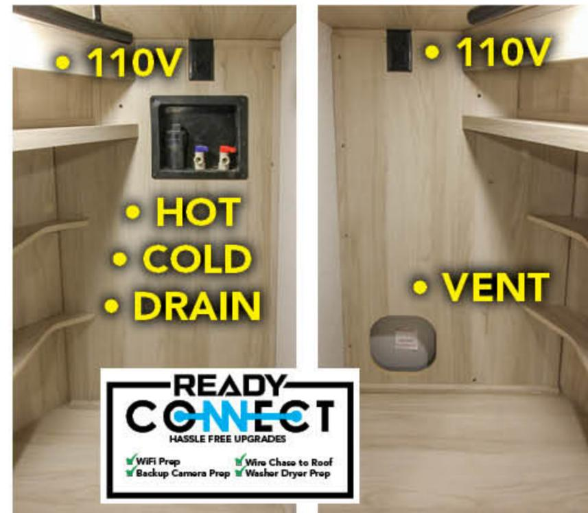
We make it easy to add a washer and dryer with dedicated locations pre-engineered to accept the washer and dryer with 110 volt outlets, color coded hot and cold water hookups, drain connection and outside vent location all ready for a quick and easy upgrade.
