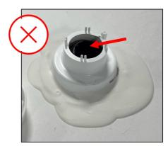
If vent pipe sits **below** the opening of the vent body, vent pipe will need to be extended to 2.5" above the roofline and vent reinstalled.
