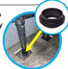
**8 PIPE CONNECTIONS** – Pipe connections that have come loose can allow odors to be present.
