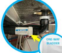
**5 P-TRAP** – Traps water in the low point to keep odors at bay. If water in the p-trap has evaporated, odors can be present.
