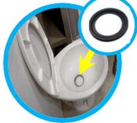
**4 WATERLESS TRAP** – One-way bladder used in tighter spaces like shower and washer. If bladder is not closing fully or is inverted, odors can be present.
