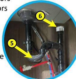
**6 AIR ADMITTANCE VALVE** – Valve that lets air in, but not out. If valve gets stuck open, odors can be present.
