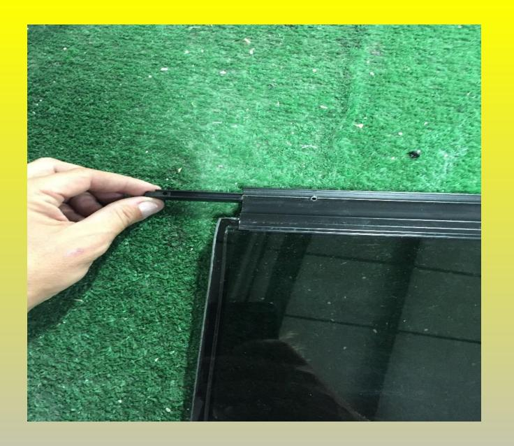
7.) Slide plunger all the way to the outside of the sash and reinsert VS latch spring
