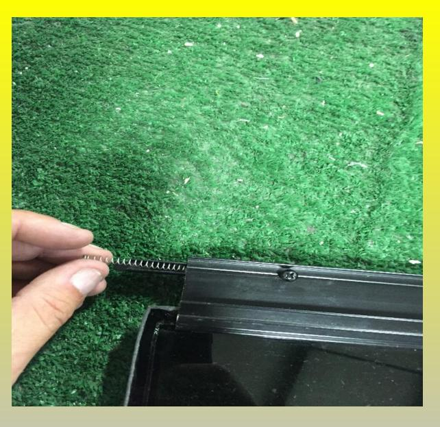
8) Line up sash back into window frame and slide sash into closed position
